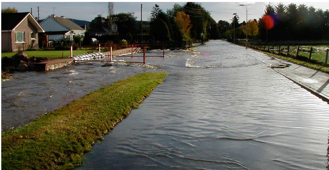
Flooding in the village of Tarland
