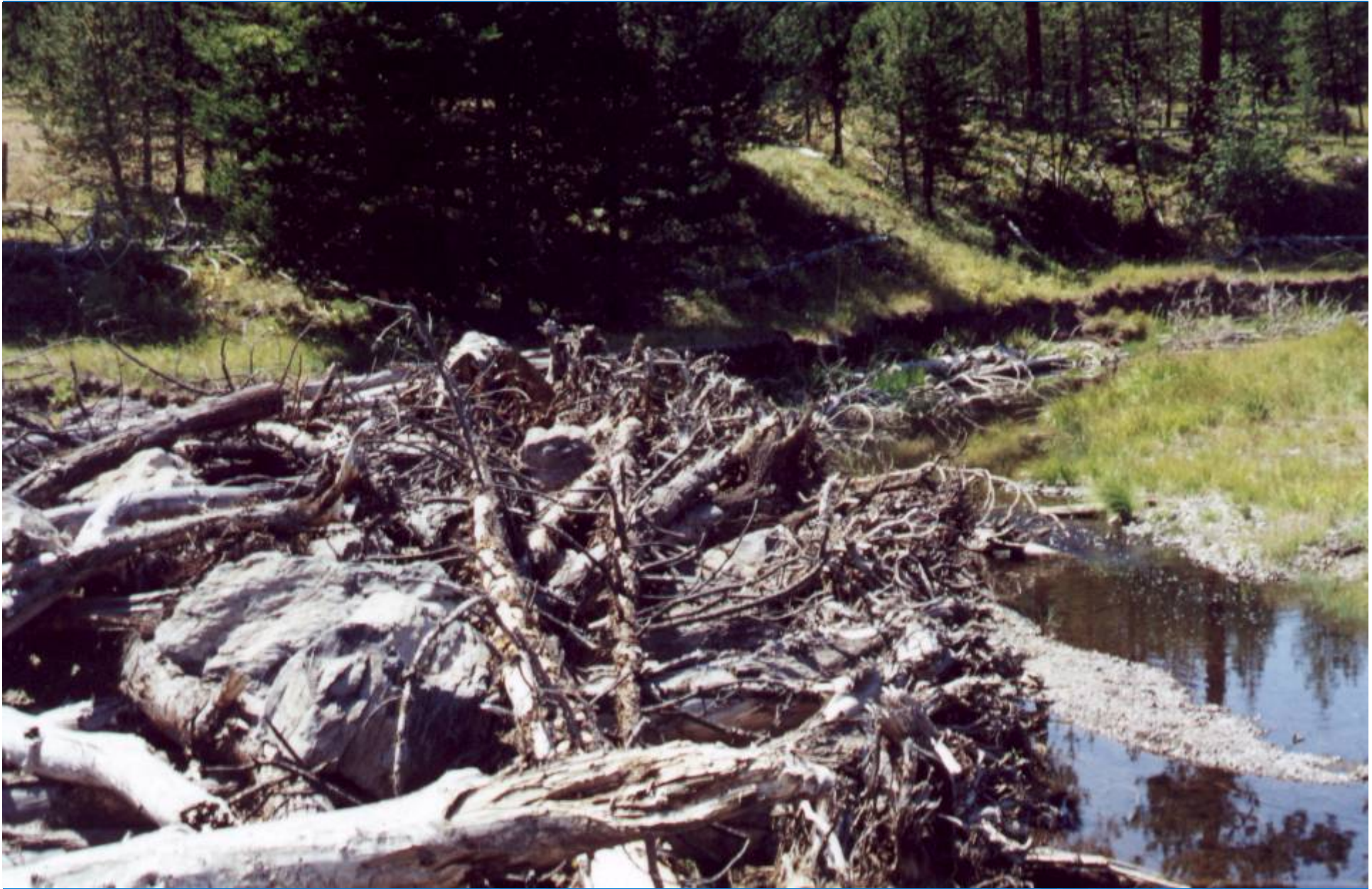
Large wood structure to shunt water into historic channel. Built in late-1990s
